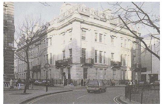
Marian Kennedy Fischer Hall - Home of Notre Dame's London Classroom/Office Building
